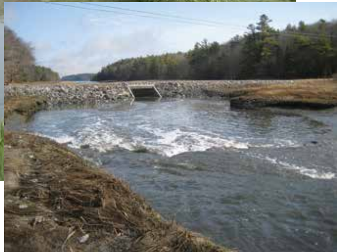
Enlarging the culvert under Long Reach Lane restores important tidal flow.
